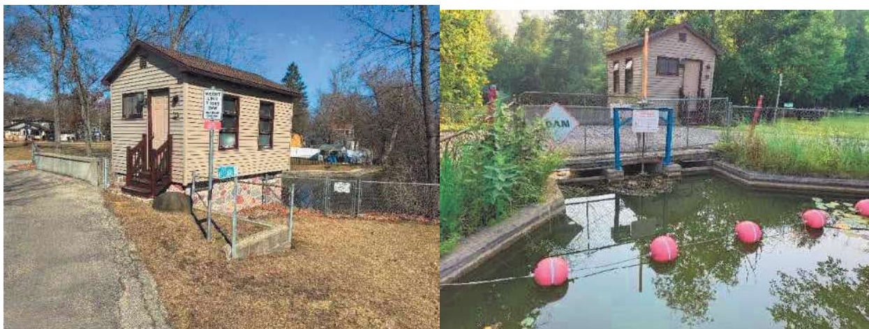
Figure 9 Wambold Storage Shed and inlet view
