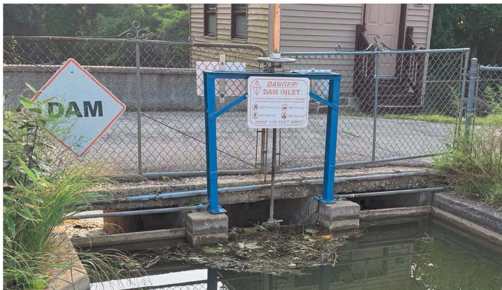
Figure 11 Notice the worm screw with crank handle for adjusting gate opening
