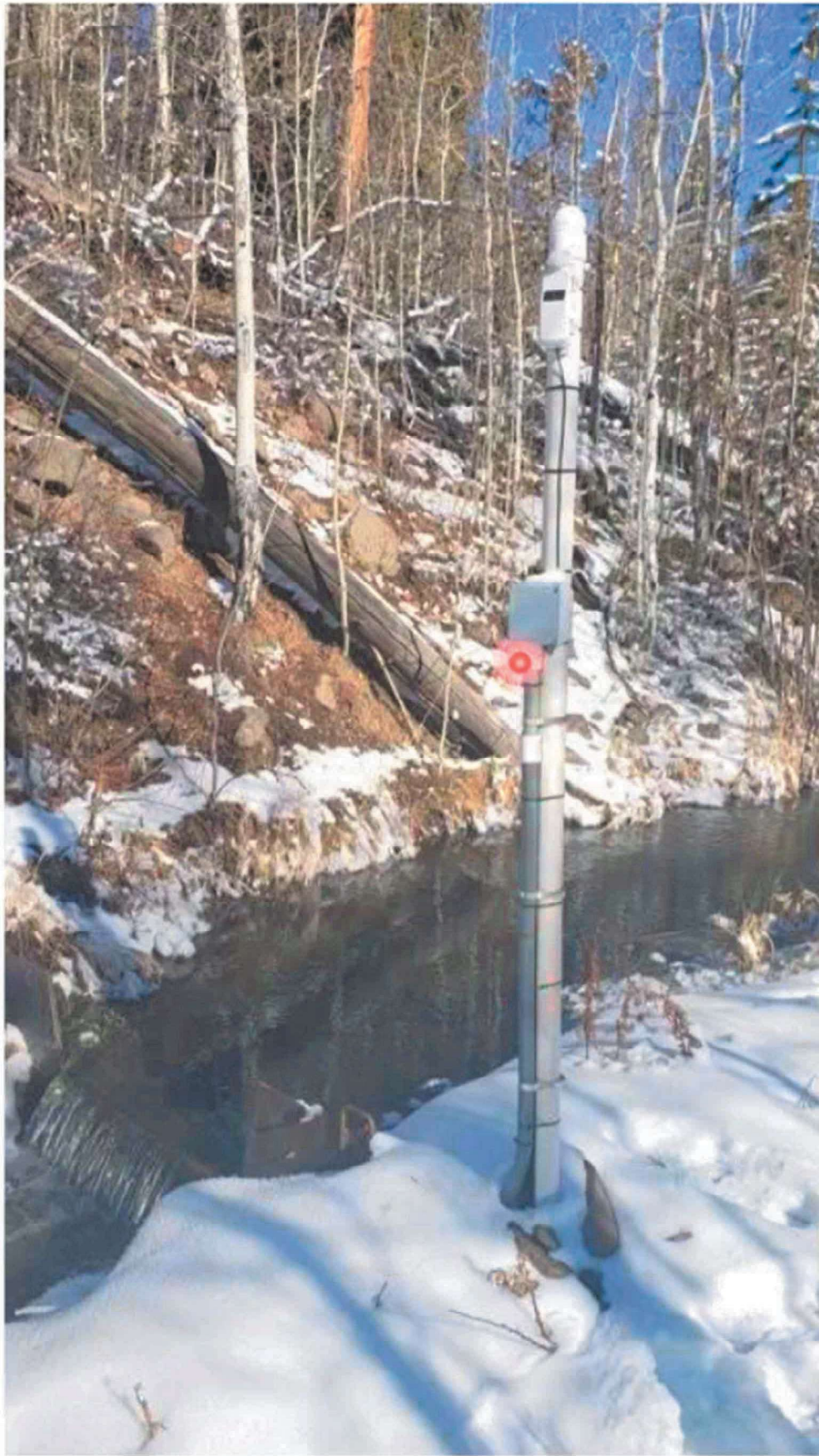
Figure 25 Example of water level gage set up with wireless mote.
