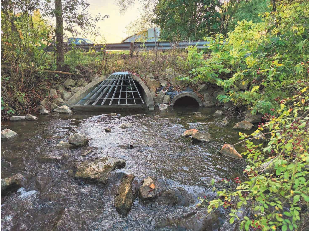
Figure 19 Kroll Outlet Culverts
