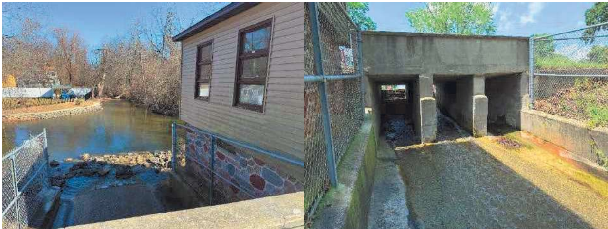
Figure 10 Notice the three spillway channels
