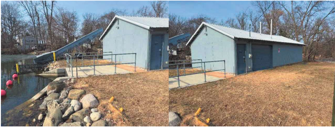
Figure 16 Notice Inlet channel
